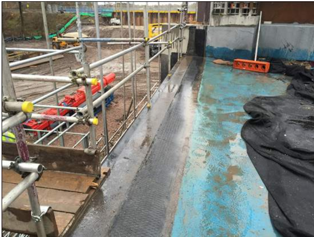
T-Mat expansion joint used on rail bridges
